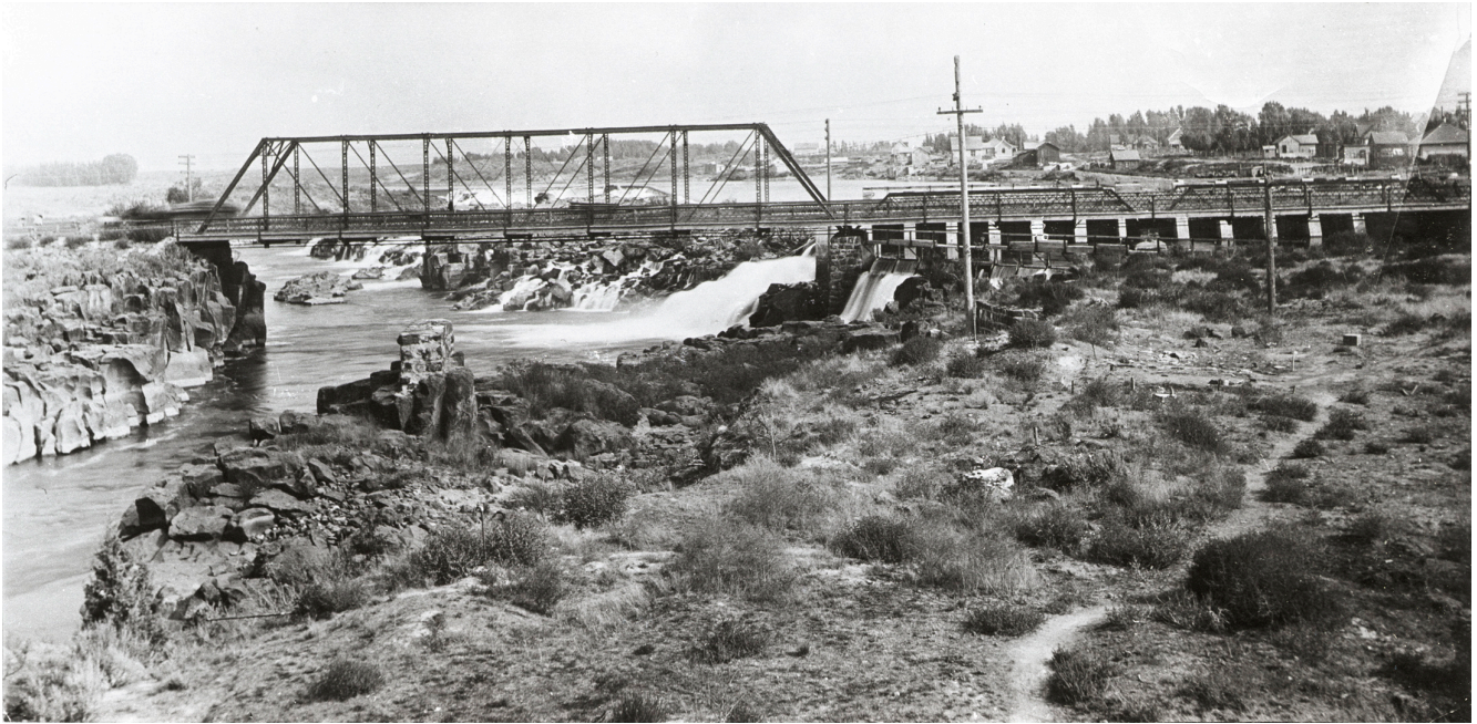
The island, circa 1920, taken from the railroad bridge embankment looking upstream. The bridge in the photo is the steel bridge that straightened Broadway. The piers from Keefer's first steel bridge are visible, one being at the base of the electrical pole. Imagine the amount of dirt that was carried in by wheelbarrow! Photo courtesy of the Museum of Idaho.
