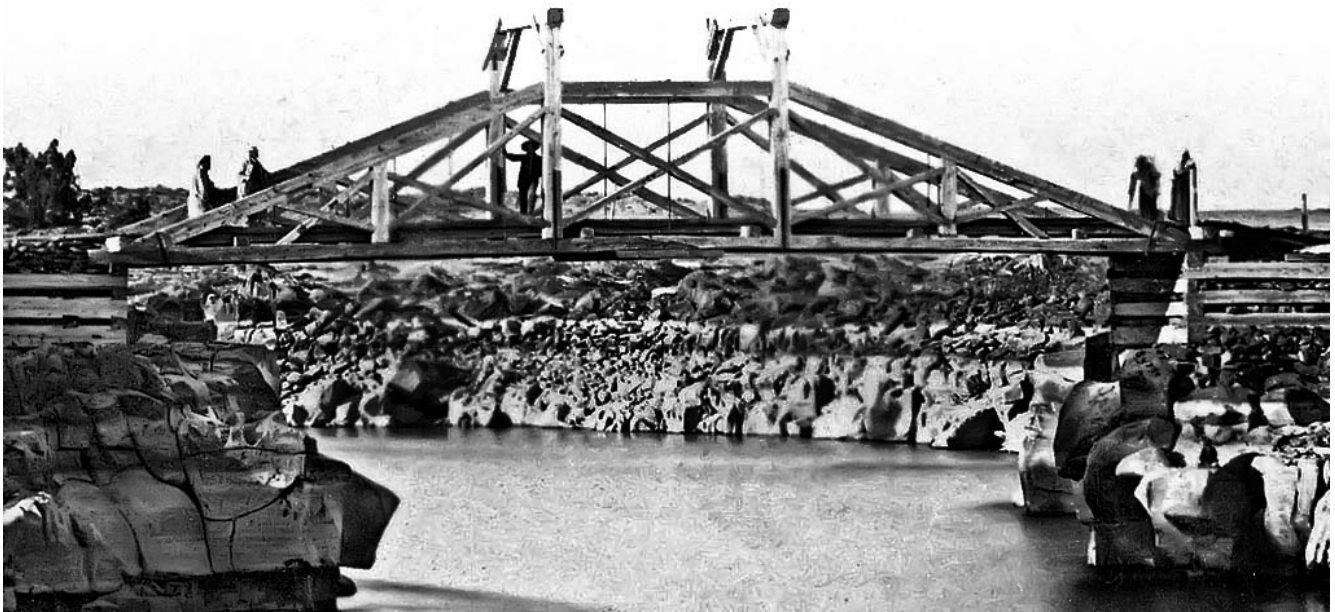
Taylor's Bridge around 1870. Note the cribs of rock which formed the piers. From the USGS files.
