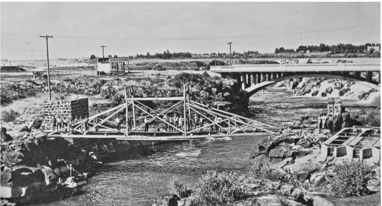
Shortly before 1934, Company F of the 116 th Engineering Division of the Idaho National Guard built this replica of the Taylor Bridge. Perhaps it was built as an exercise for the engineers, or perhaps it was built in connection with a celebration of an anniversary of the bridge or the Golden Jubilee of the Post Register Newspaper in 1934, a huge event. It is obvious
